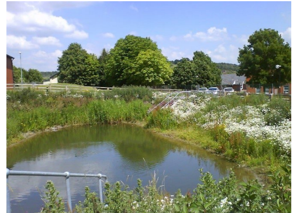
Figure 20. Typical Drainage Attenuation Pond
