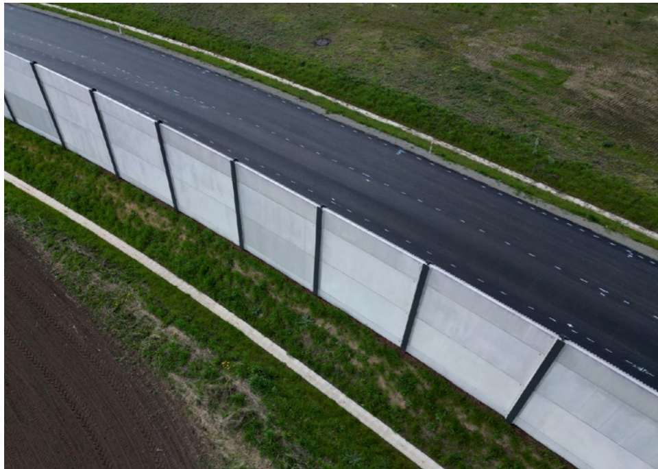
Figure 17. Noise Barrier Wall
