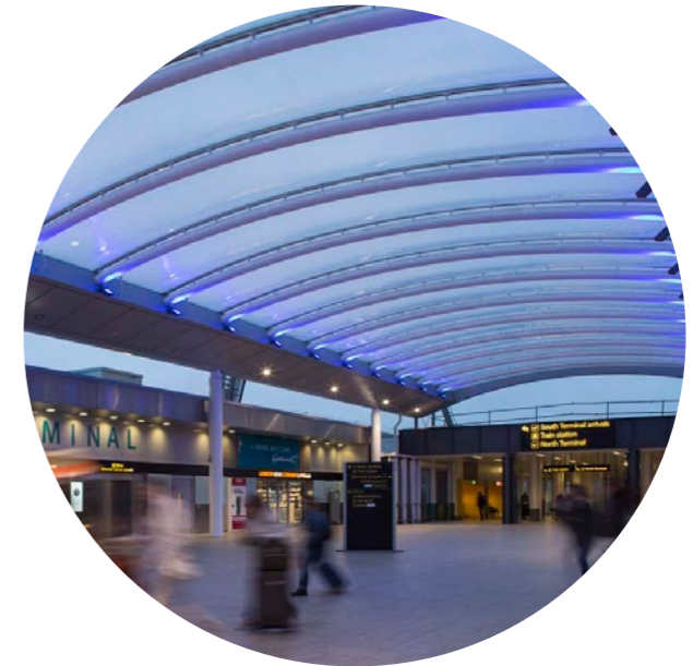
Figure 5. Built Form: Gatwick South Terminal Forecourt Consider Gatwick’s existing fabric to create a coherent development
